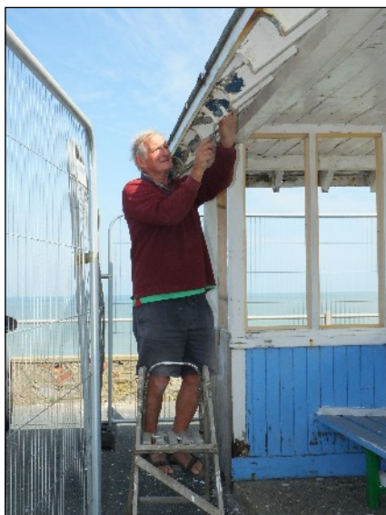
Mike Wiseman at work restoring the shelter - July 2019
